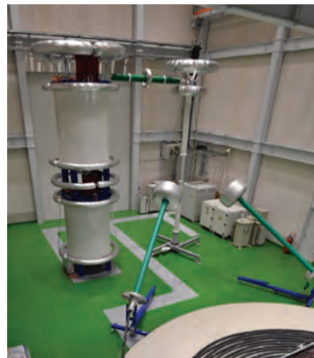
Highly Aged XLPE Power Cable Deterioration Test Facility
