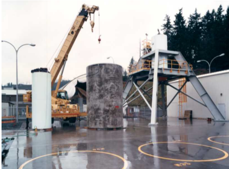
Example - Ventilated Dry Cask System
