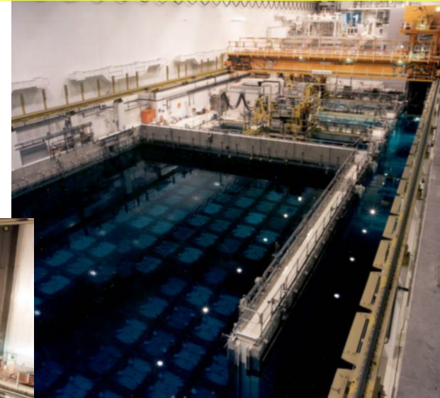
Fuel Handling Plant – Magnox & AGR
