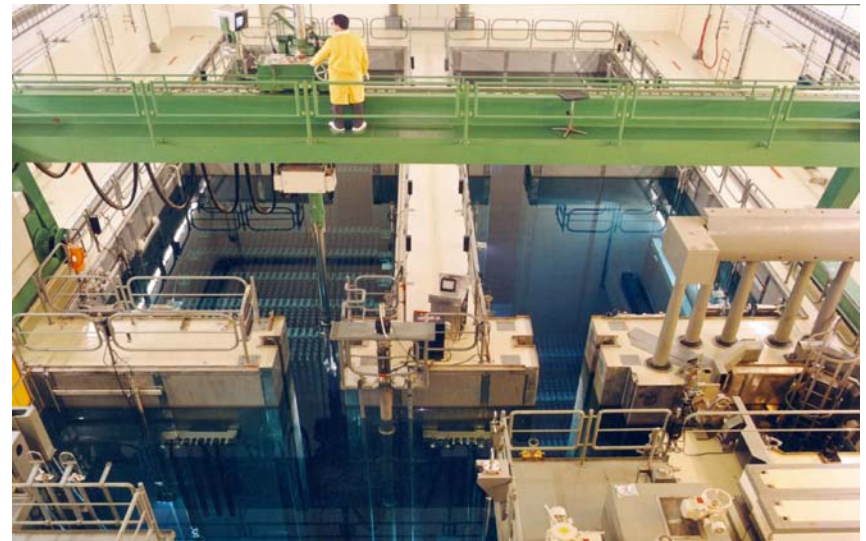
Panoramic view of the four pools of the building 2, the monitoring pool (down) and the bridge. ANPP I.
