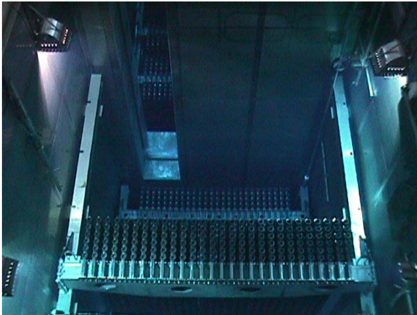
Hanger loaded with fuels in the pool (upper level). Below the lower level (level 1)
