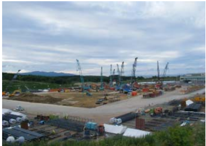
Fig.1 status of construction (Shooting date: September 10, 2010)
