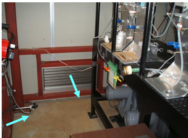
Air Inlet of Test House
