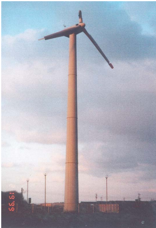
Fig.1 Damage of wind turbine blade due to lightning
