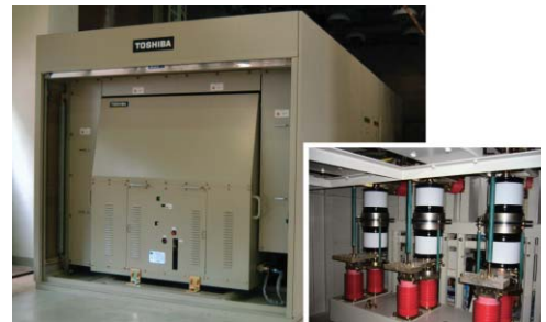
Backup circuit-breaker system
