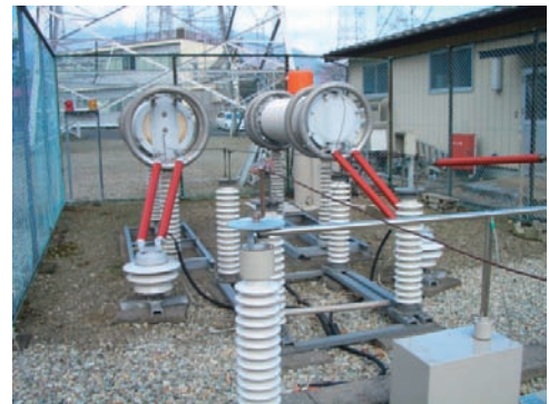
DC voltage generation circuit
