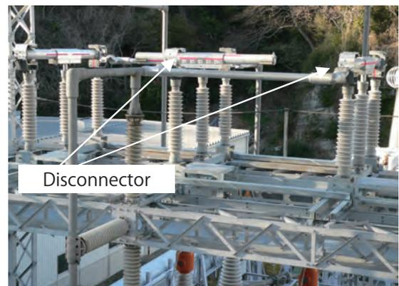
Photo 2: 115kV Horizontal Break disconnector (3-unit interlock operation)
