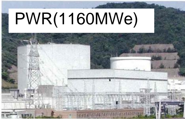
Tsuruga Power Station Unit 2 Japan's first advanced standard pressurized water reactor
